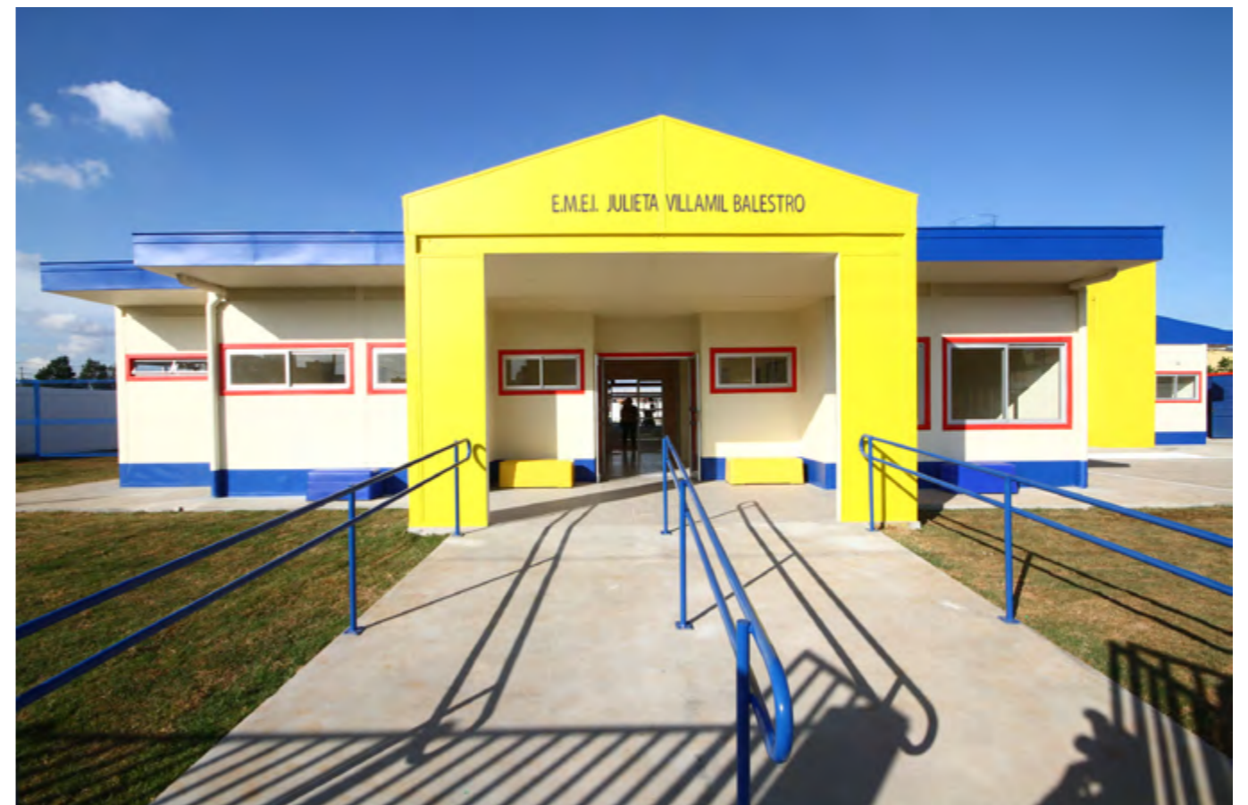
School Constructed with Wall System
